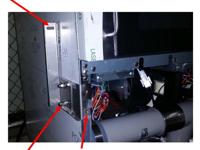
STEP 4: ONCE THE LOCATION IS FOUND. MARK WHERE THE BRACKET WILL BE MOUNTED TO THE CABINET SIDE AND DRILL A .145 DIA HOLE. USE THE SUPPLIED CABINET SCREWS TO SCREW THE BRACKET IN PLACE.
